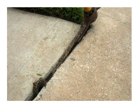
2. Fill gap with flexible polyurethane foam backer rod. Rod should be snug; if it is loose, twist two rods together to make a larger diameter.
