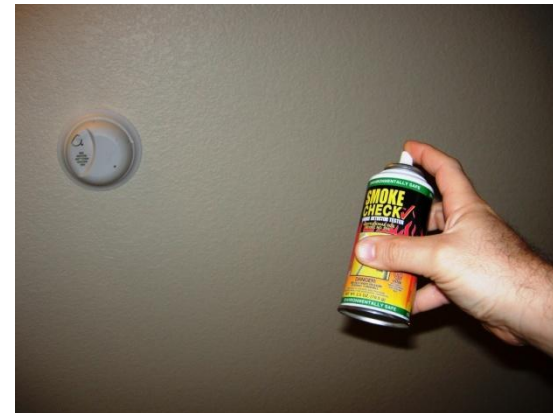
Testing the Smoke Sensor
