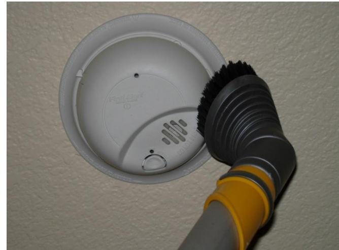
Cleaning the Smoke Alarm
