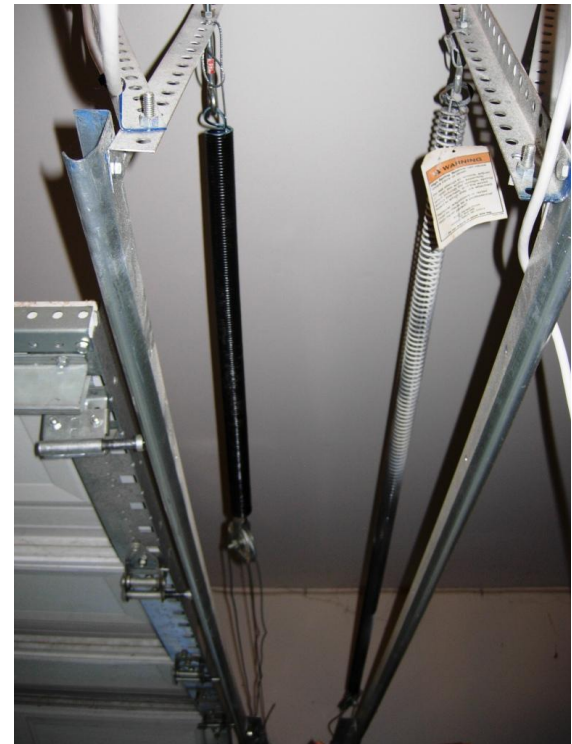
In-line extension springs
