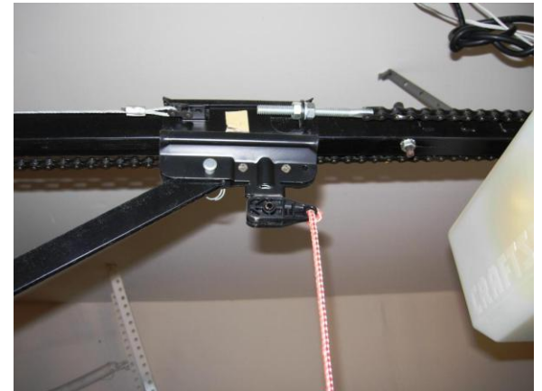
Flip lever back horizontally to re-connect door to opener
