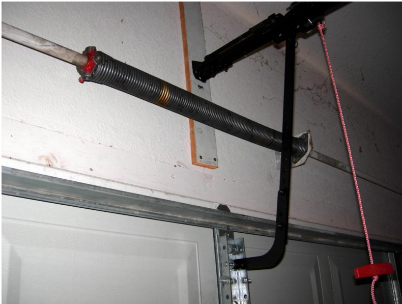
Overhead torsion spring
